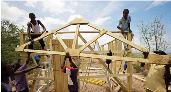
5.11 Timber frame construction, Leogane/Haiti 📷 Cordaid Haiti.
