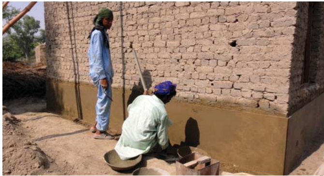
5.6 Plastering to protect external walls from flood risk, Pakistan IOM Pakistan.
