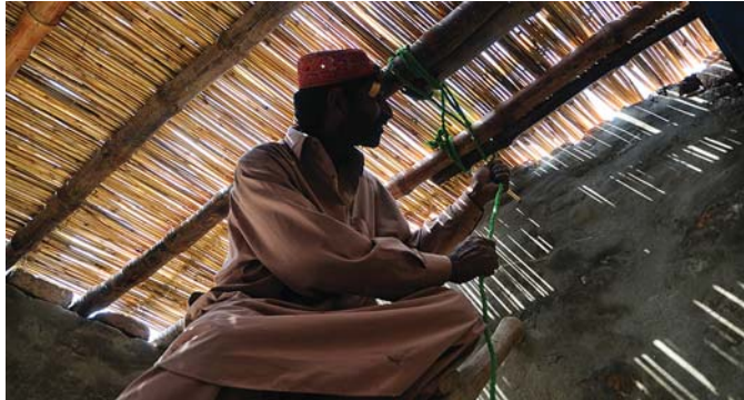
5.13 Bamboo roof structure, Pakistan 📖 Usman Ghani/IOM Pakistan.
